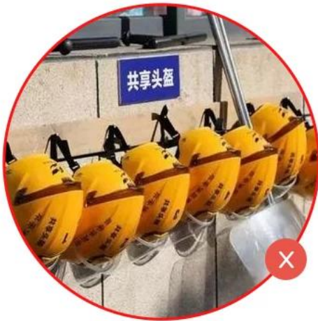
Helmets hang with rope disorderly, easy to drop and crash
